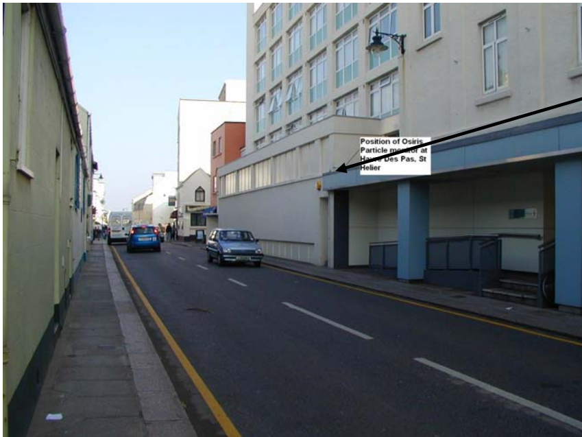
Photograph 3: Position of the Osiris unit at Havre Des Pas
